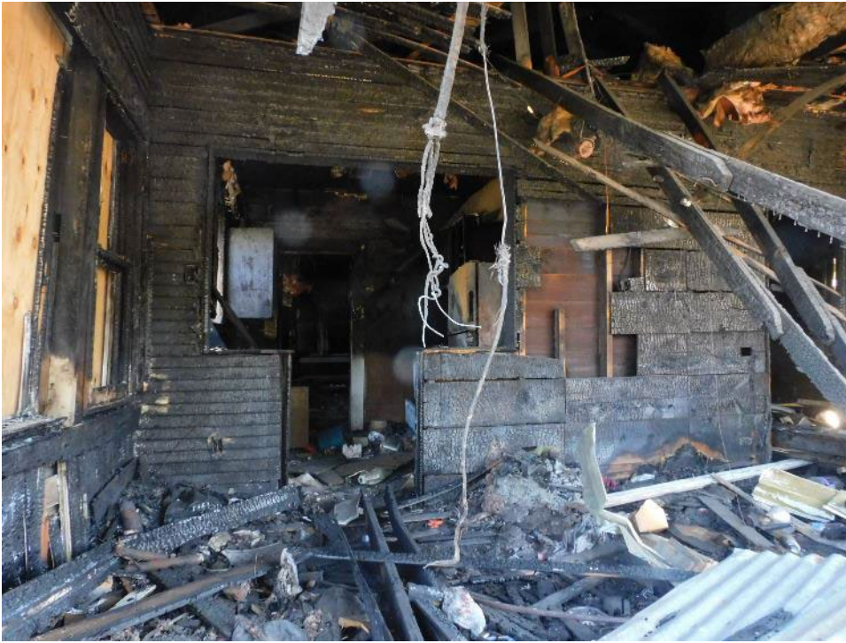
Photo 7, Interior, damage to walls and framing.
